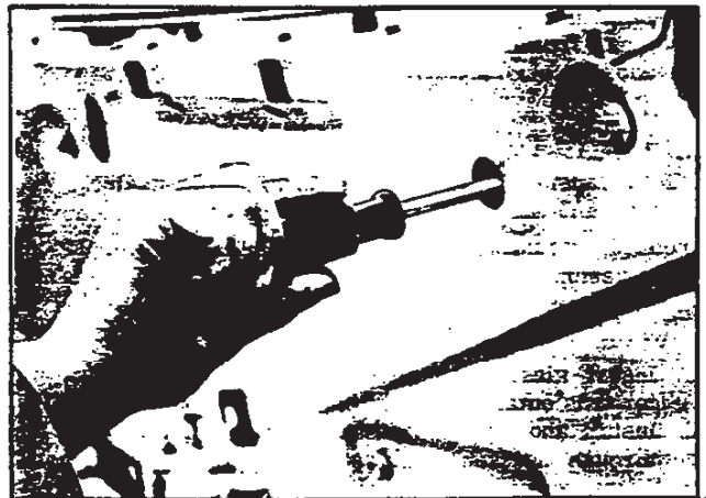
Fig. 28—Removing Sash Screws
