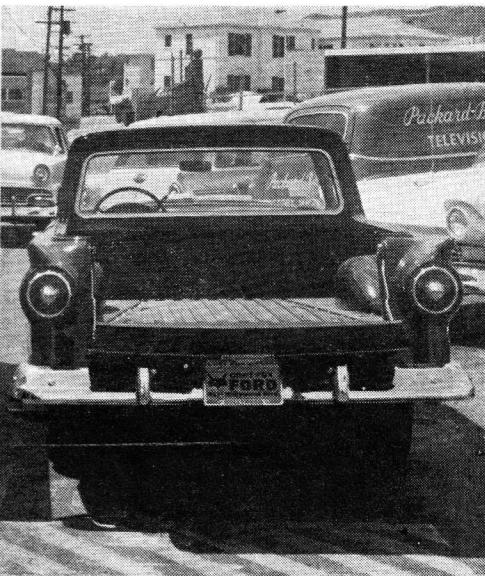
In styling, the Ranchero is much lower than the  $\frac{1}{2}$ -ton Ford F-100 pickup and doesn't have as many cubic feet of bed but width of tailgate opening is the same.
