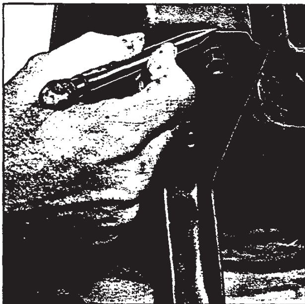
Fig. 37—Marking Hinge Position
