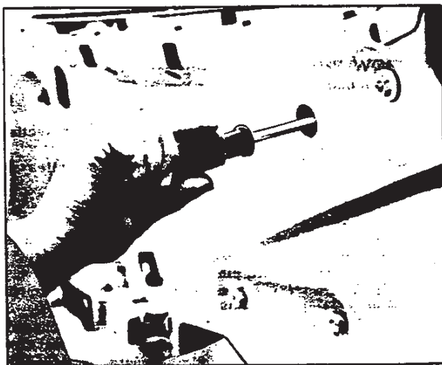
Fig. 24—Removing Sash Screws
