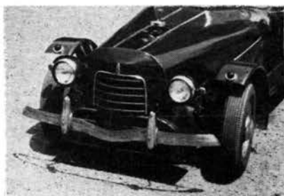
Stripped sportster shows typical framework of tubing on chassis. Usual basis for cars is 1932-40 Ford, which may be modified by shortening the wheelbase.
