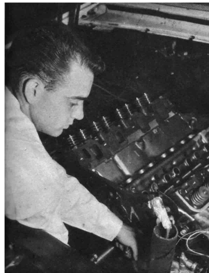
Out comes the smog-control paraphernalia. The manifold is plugged up, too.
