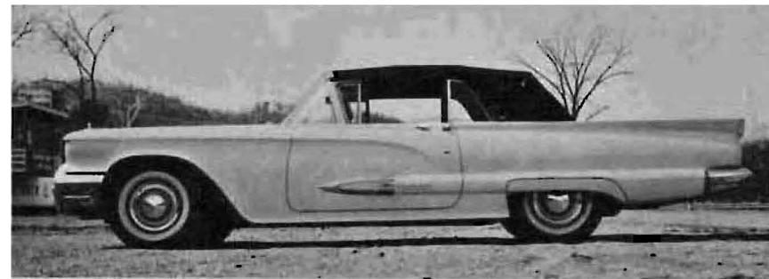
Side view of '59 'Bird shows close-coupled passenger compartment contrasted with fairly long hood and trunk. Integral body frame construction permits low silhouette with good headroom.
