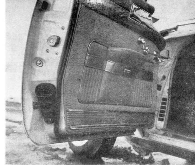
WARM AIR for rear seat heater is ducted through the doors, as can be seen here. This is making the most of waste space, in the lower portion of the doors, which is most generally left unused.
