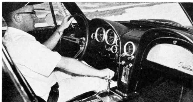
As in any well planned sports car interior, everything proved easy to reach, read, and see. Comfortable buckets give good support, adjust for rake. Sturdy shift lever is well located.
