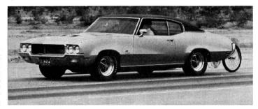
profile tires are optional. The G78's on the rear did aid initial acceleration, though the relatively high stall speed of 1500 rpm can cause the rear wheels to slip if full stall is exercised. Driving out from a lower speed, around 1000 rpm, resulted in a more constant lowend pull and shorter time on the clocks.
